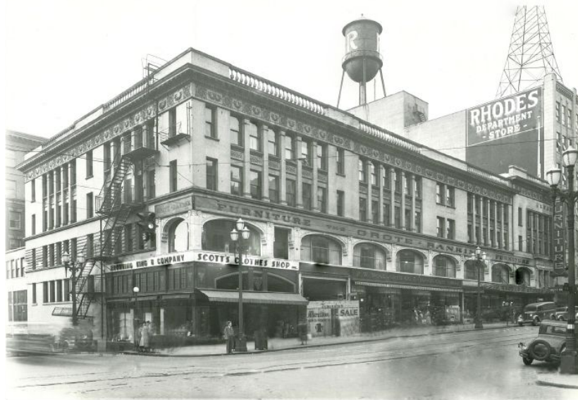
54. Arcade building, Seattle, 1932.
